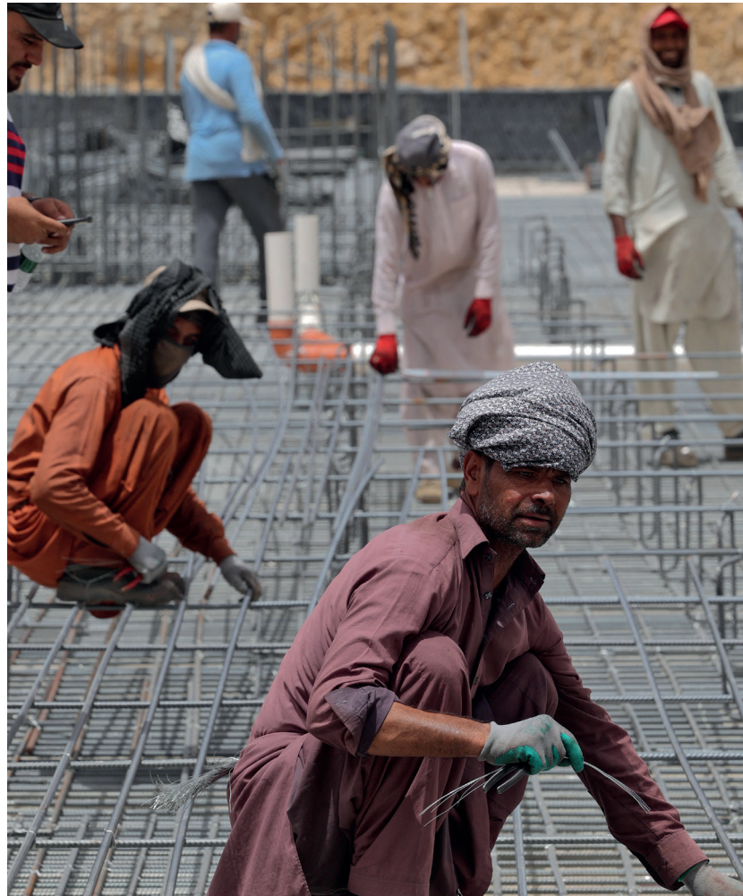
Labourers work on a steel mesh at a construction site in Saudi Arabia's capital Riyadh on May 23, 2022 during a heat wave. © FAYEZ NURELDINE/AFP via Getty Images
